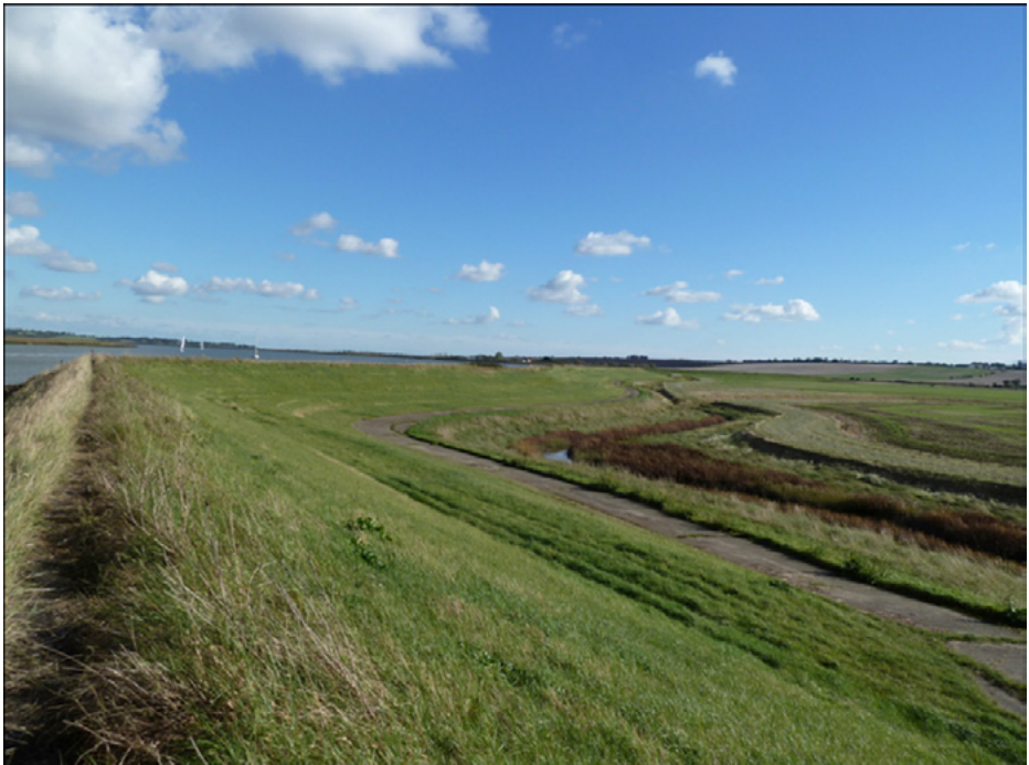
Photo 2: South Fambridge waste filled flood embankment.
