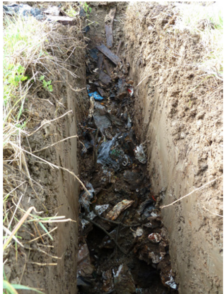
Photo 1: Historic landfill waste in situ in Hadleigh Marsh waste filled embankment.
