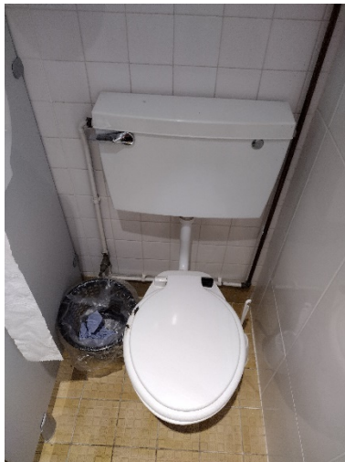
Figure 12: Examples of the one -stage toilet tanks in East Block
