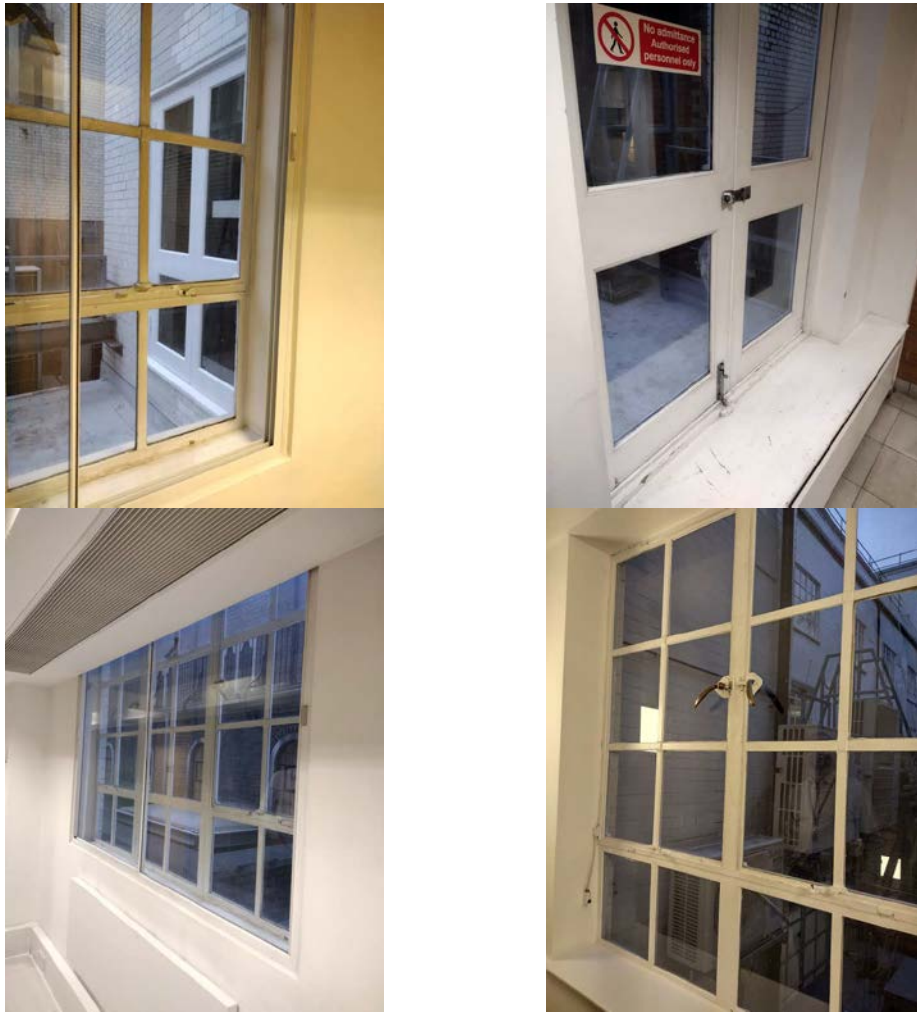
Figure 2: Examples of windows/doors in buildings
