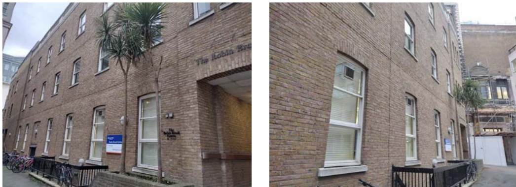
Figure 1: Examples of outside walls in buildings of the Robin Brooke Centre
