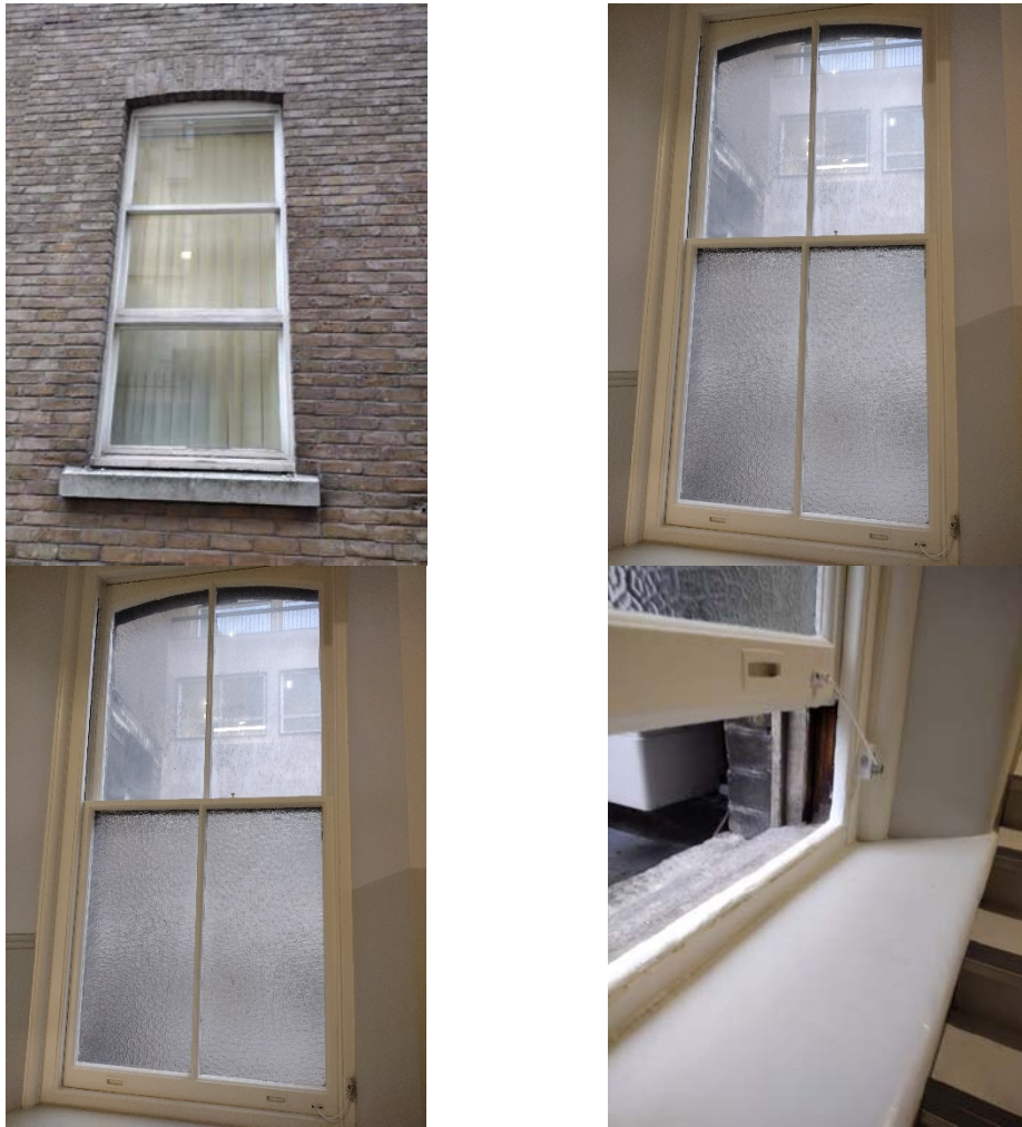
Figure 2: Examples of windows/doors in buildings of the Robin Brooke Centre
