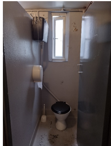
Figure 12: Examples of the one -stage toilet tanks in East Block
